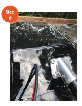
Thread wires from roof to the interior of the tent.
