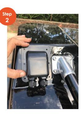
Place the entry gland and drill the first hole, then insert the rivet to hold it in place (do not compress the rivet yet).
